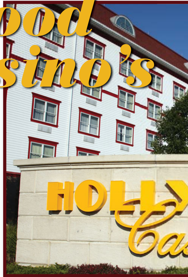
The Hollywood Casino video surveillance project involved connecting the system from the main building above to a new "superboat" (inset, upper right).
