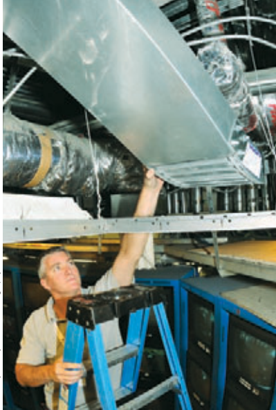
TSI's Thomas Swankosky, who has been involved in more than 100 casino system projects, installs the raceway enclosing the cabling from the server room to both the security and surveillance control rooms.
